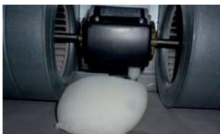
Duct Air Treatment in Ducted Unit
